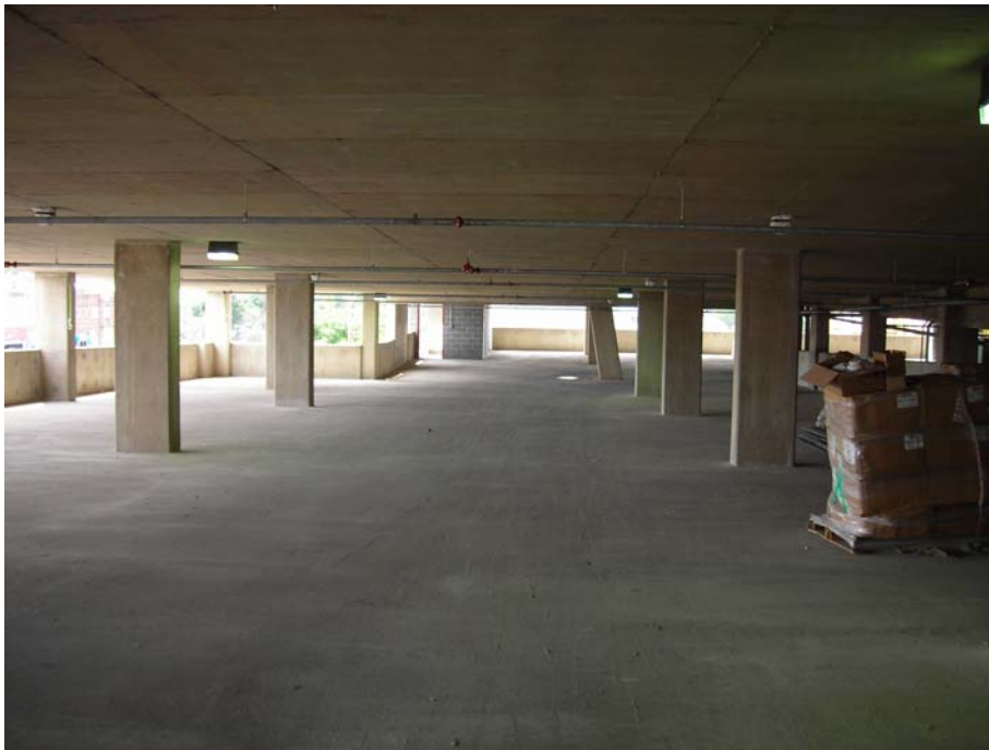
Photo 6: Interior View of the parking garage.
