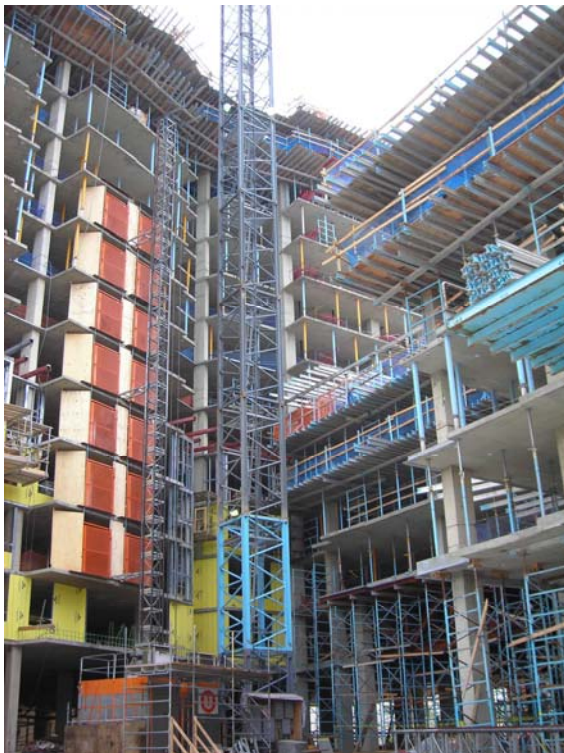
Photo 4: Partial view of the inside corner between the Southwest elevation and a small portion of the West elevation.
