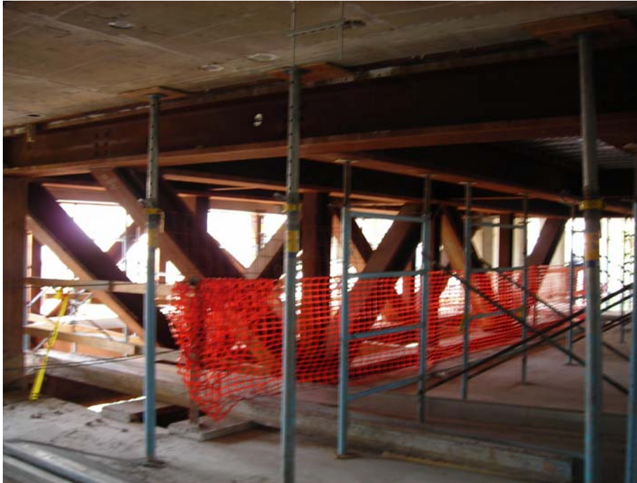
Photo 7: Interior view of pedestrian bridge steel structure.
