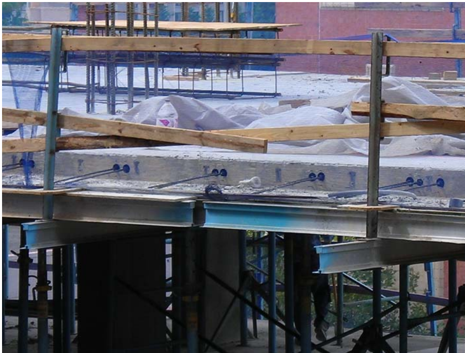
Photo 10: View of post-tensioning cables prior to jacking force application.
