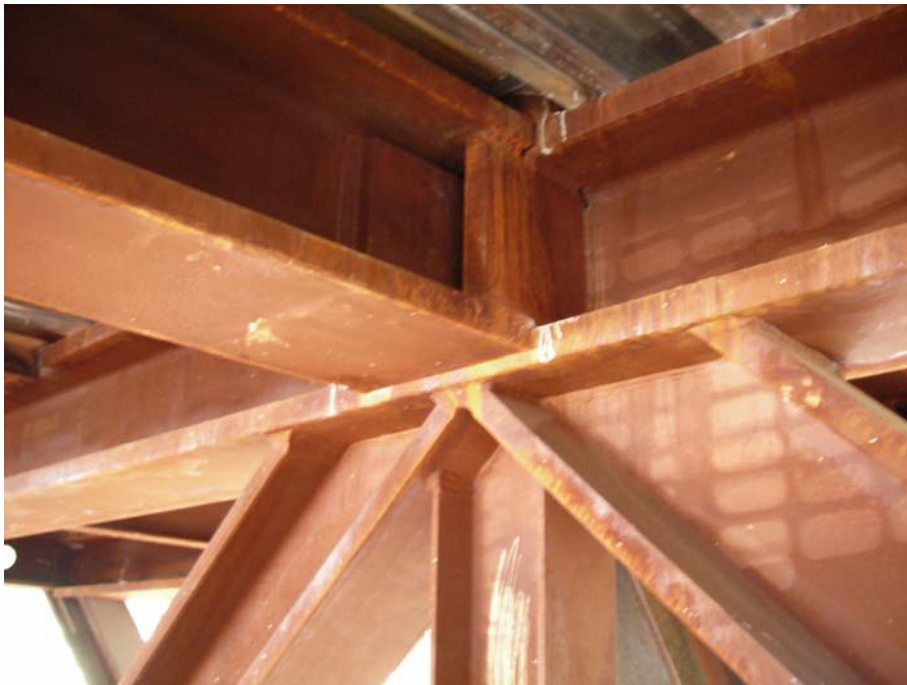
Photo 8: Typical full penetration welded connection of the bridge truss structure.
